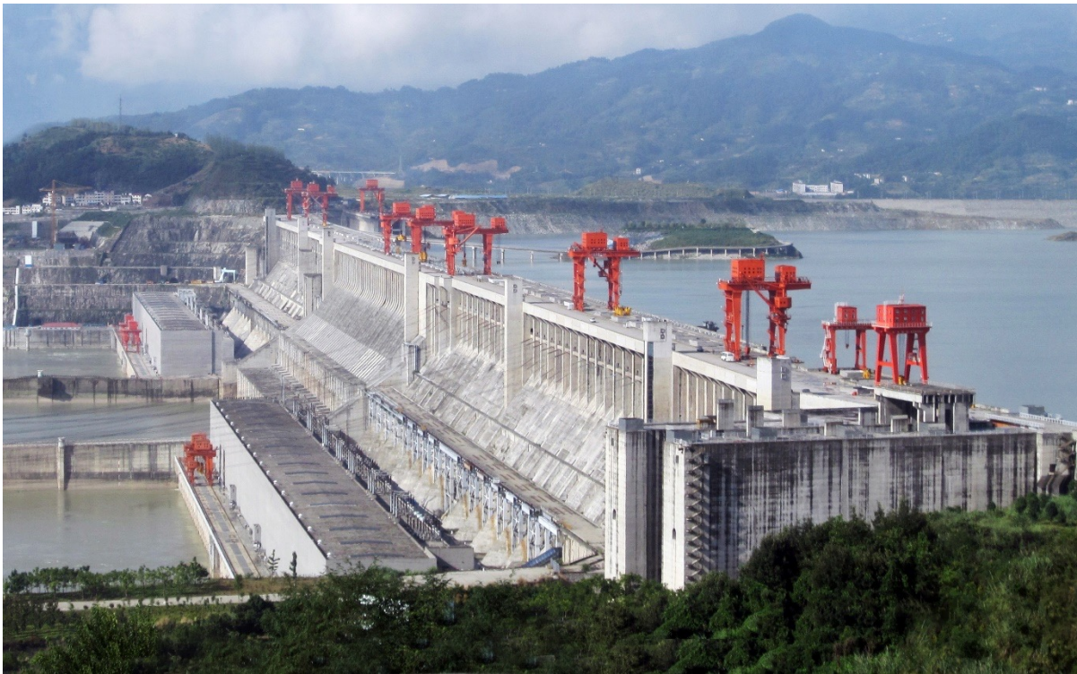
Three Gorges Hydro Electric Dam in China (Credit: Le Grand Portage licenced under CC BY 2.0, [205])
