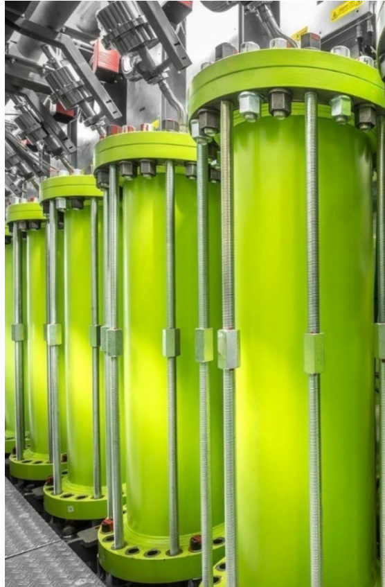
Flywheel system for wind farms and public transport (Credit: STORNETIC GmbH [212])
