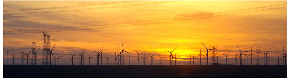
Figure 1-32: The onshore Gansu Wind Farm in China.
