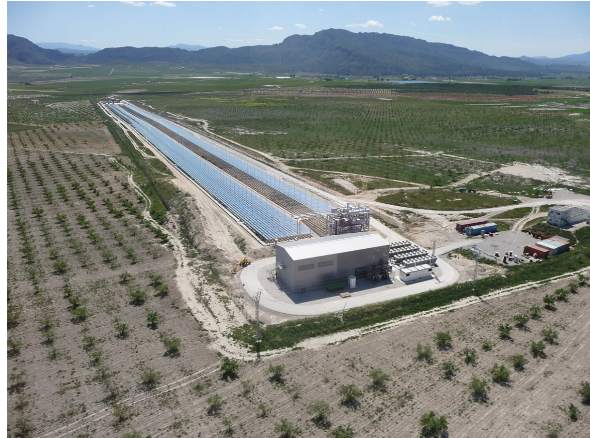
Figure 1-17: Linear Fresnel reflector technology at Puerto Errado 1 solar thermal power plant, Spain.
