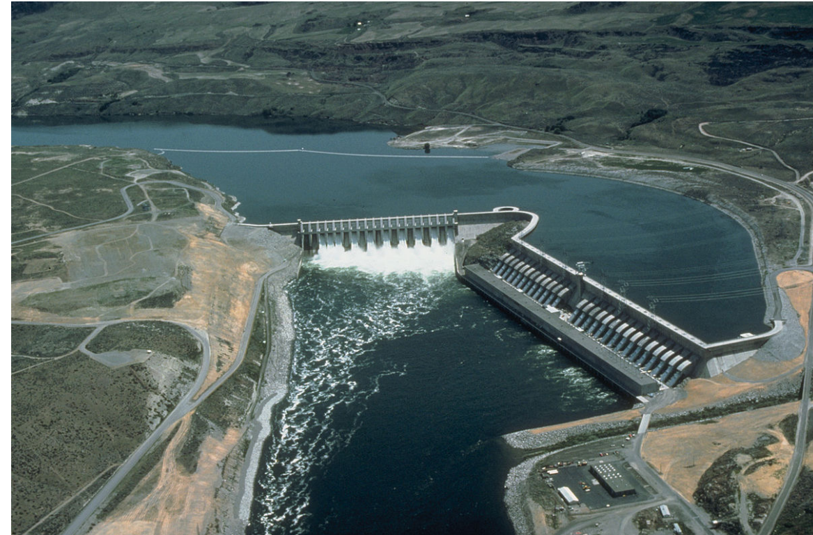
Figure 2-25: Chief Joseph Dam, a run-of-the-river plant in Washington, USA.
