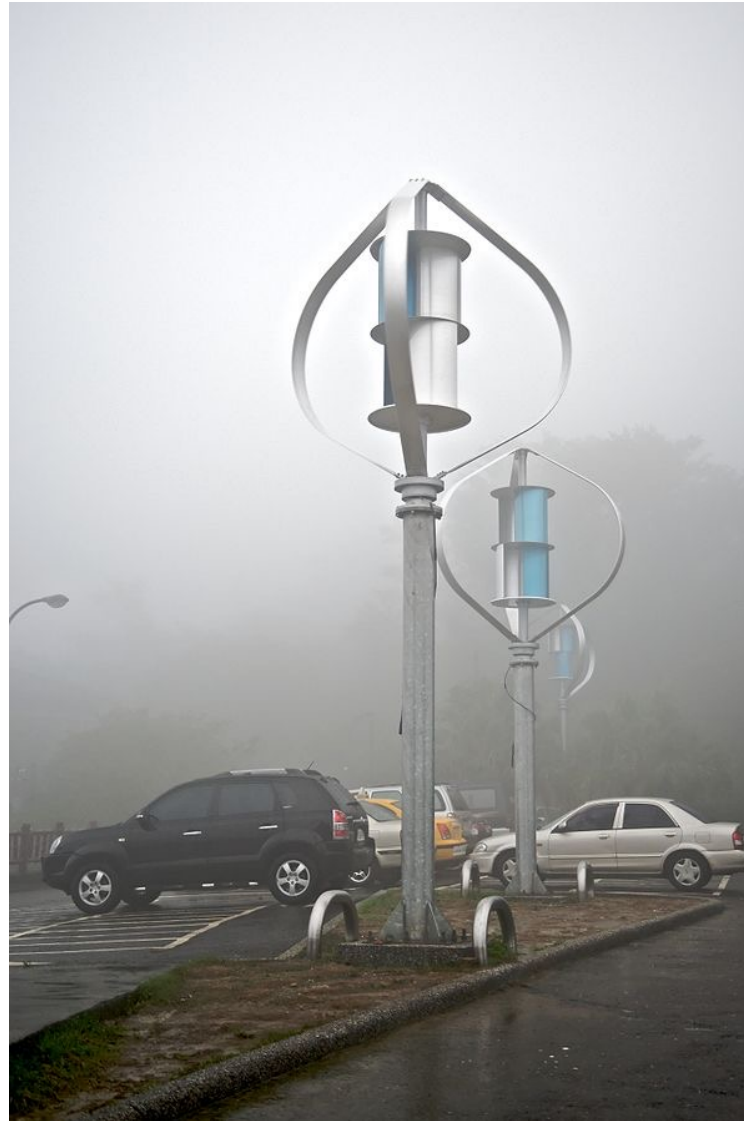
Figure 1-31: Combination turbines of Darrieus and Savonius designs in Jinguashi, Taiwan.
