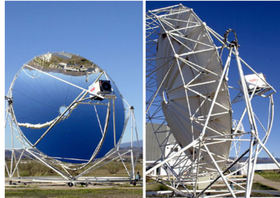
Figure 1-18: EUROdishes at Plataforma Solar de Almeria.
