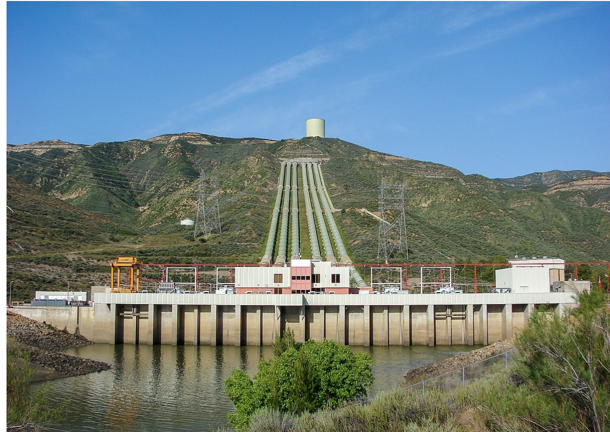
Figure 2-23: The Castaic Pumped Storage Plant, USA.
