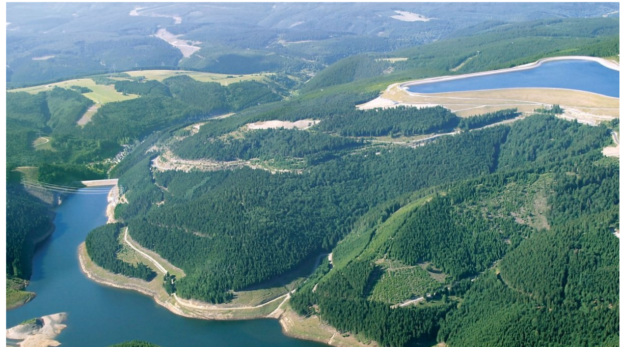
Goldisthal Pumped Storage Hydro Electric Dam in Germany (Credit: Voith under Written Permission, [206])
