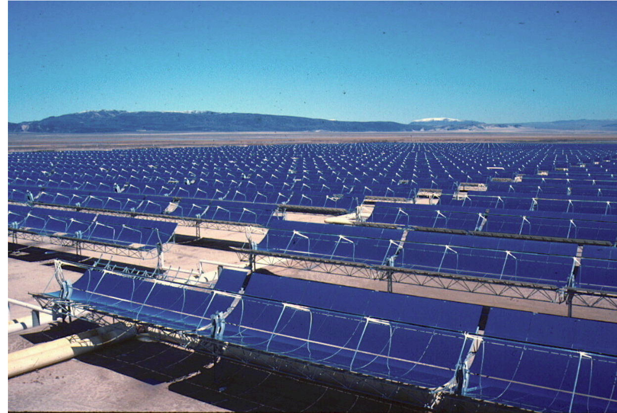
Figure 1-15: Parabolic troughs at the SEGS plant, USA.
